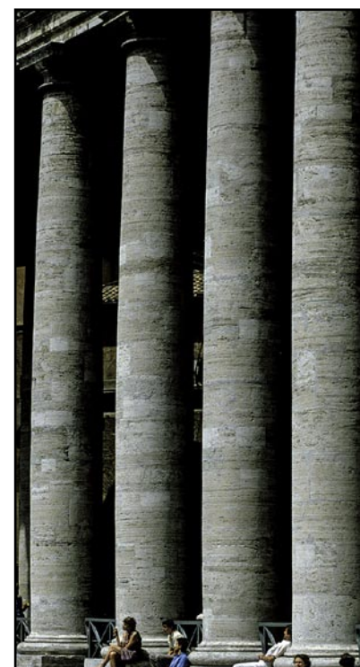
Figure 29: Columns of banded travertine around St Peter’s Square in Rome, fashioned from rock that was sourced from quarries east of the city.
