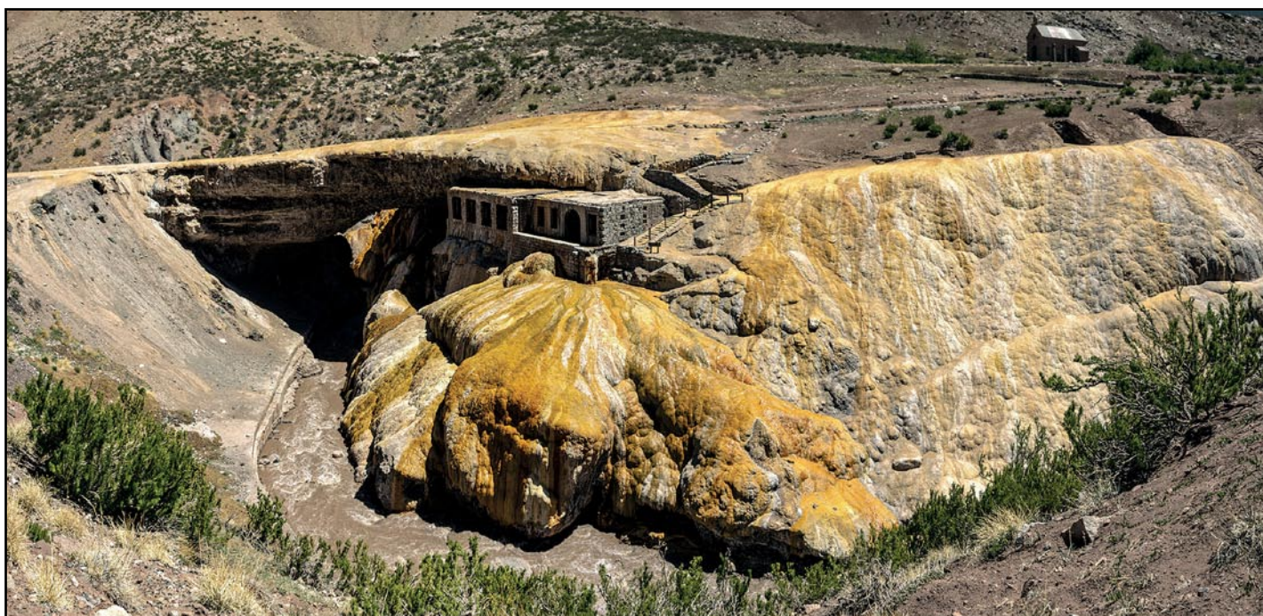
Figure 34. Puerta del Inca (the Inca Bridge), formed of travertine that has been undermined by the Rio Mendoza in the Argentine Andes.
