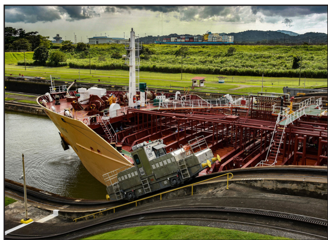
Figure 17. A ship and one of its guiding mules in the Miraflores Locks; in the background, a container ship on its way to the Cocoli Locks is in the high-level canal retained behind the Borinquen earth barrier.
