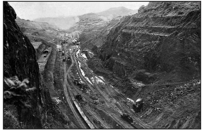
Figure 6. Excavations in the Culebra Cut during 1913, looking north from Contractors' Hill, with rock terraces in Gold Hill on the right, the toe of the Cucaracha Slide lower right, and the lower slopes of the West and East Culebra Slides in the distance (photo: U.S. National Archives).
