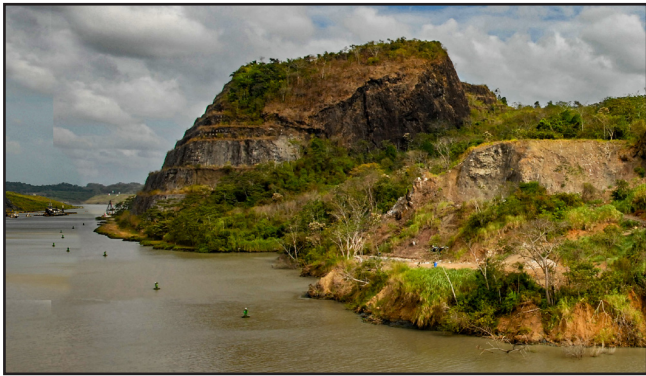
Figure 14. The distinctive terraced rock face on Gold Hill, with the broken ground of the Cucaracha Slide on the right, still creeping into the Canal within the Culebra Cut.
