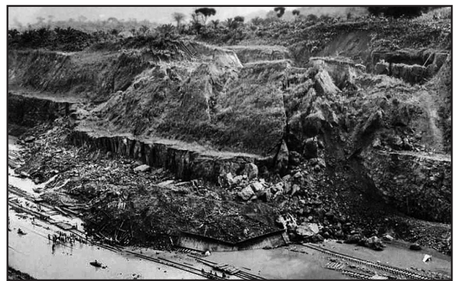
Figure 9. Slab failure into the shallow part of the canal trench between the Culebra Cut and Gamboa. A mass of strong volcanic rock has failed in front of a low-angle oblique fault, and has pushed underlying clay up into the floor of the excavations (photo: U.S. National Archives).
