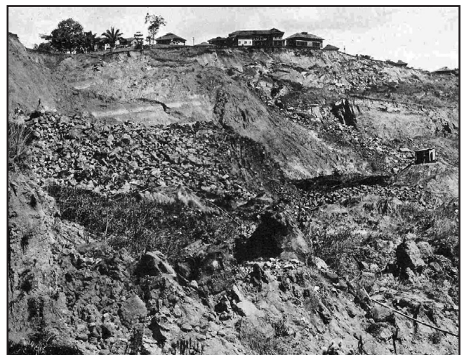
Figure 13. The West Culebra Slide expanding headwards and progressively undermining the houses of Culebra village (photo: U.S. National Archives).
