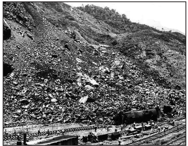
Figure 8. One of the many landslides into the Culebra Cut during the work of excavation (photo: U.S. National Archives)
