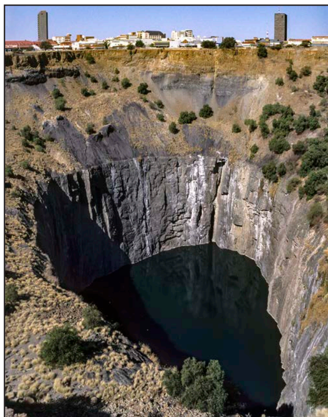
Figure 1. The Big Hole, in the centre of Kimberley; dug by hand into the Kimberley pipe, it was later undermined by block caving, and then flooded to water table.
