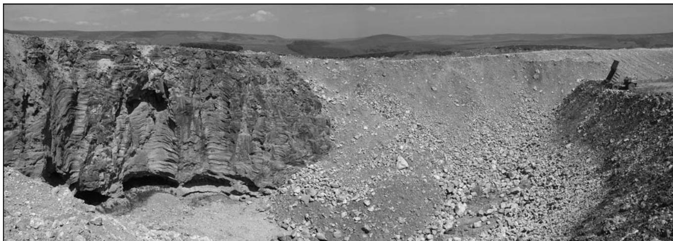
Backfilling the open pit in summer 2007. The tipper is on the fill at its intended level, which will finally reach a slope down to the foot of the face with the solution features.
