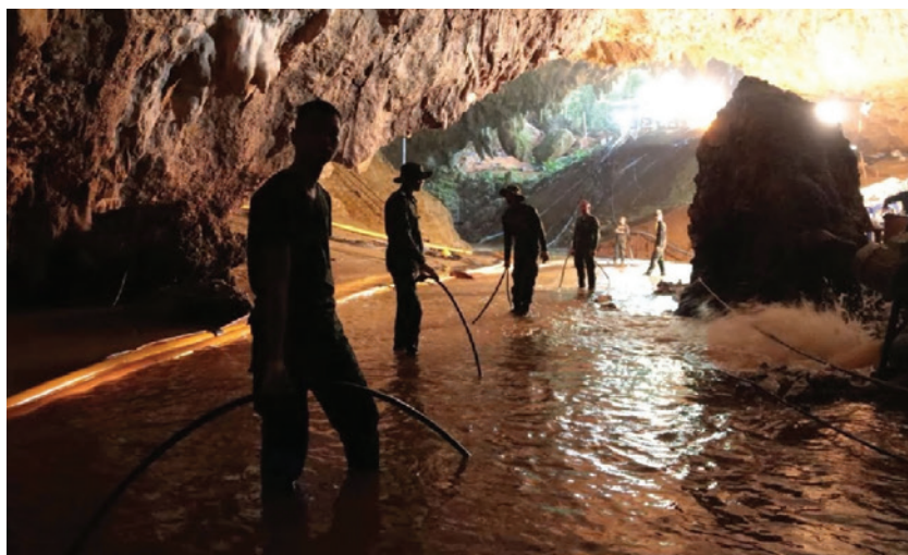
Fig. 8. Thai soldiers laying pipelines from the pumps in the large entrance passage of Tham Luang. (Image: Thai Navy.)
