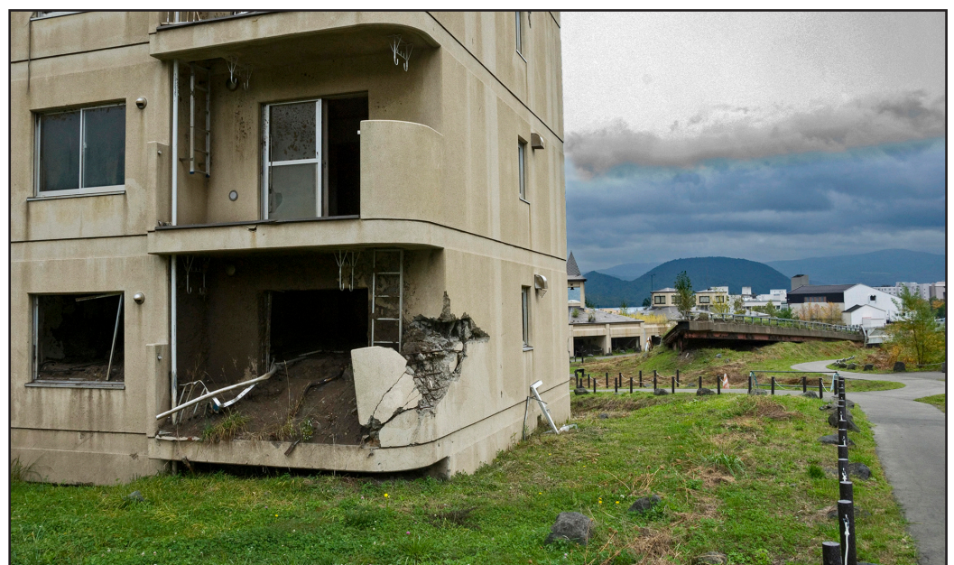
Figure 5. The corner of the one remaining block of the Saguragaoka apartments, with the ground-floor flats almost buried and the upstairs balcony that was hit by the bridge carried down by the lahar; the bridge deck can be seen on the right, where it came to rest, on a mound of debris just beyond the footpaths.
