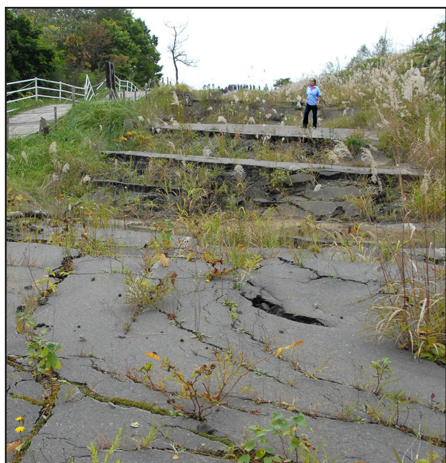
Figure 8. An old road broken by a series of fault scarps that developed during growth of the Nishiyama cryptodome.
