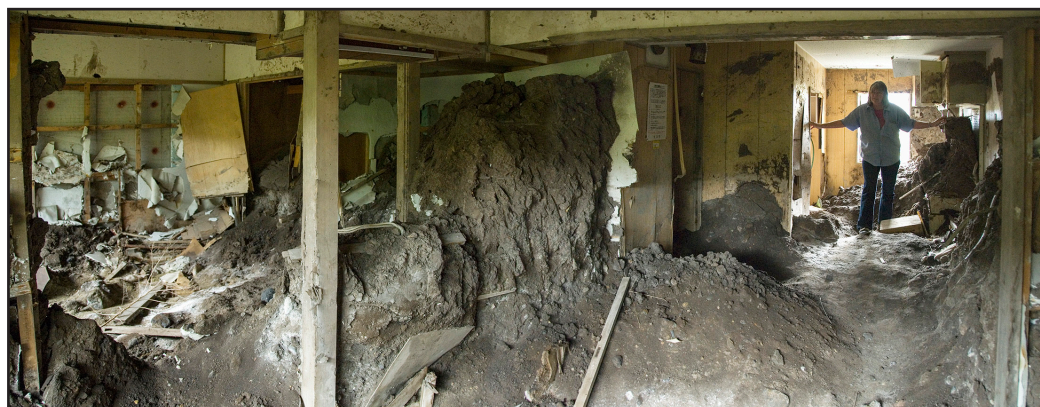
Figure 7. Rooms choked with lahar debris inside the Saguragaoka block that has been preserved.
