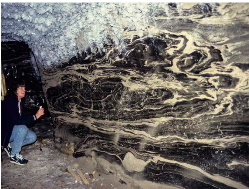
Fig. 10. The wall of the first gallery in the Tuk village ice cellar. Glass-clear ice appears black because it reflects no light at all, and the convoluted white bands are fine quartz sand. Giant hoar frost lines the ceiling where warm air accumulates from visitors' breath, and the floor is covered with fallen ice crystals and sand.
