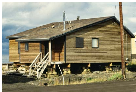
Fig. 11. A typical house in Tuk, raised on wooden blocks to ensure that no escaping heat thaws the permafrost foundations.
